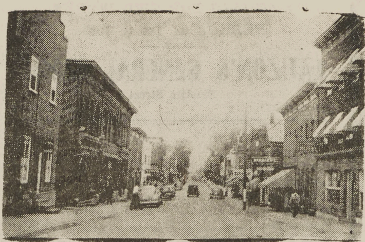
MAIN STREET TODAY — Alexandria's main street looking north from the St. Paul street intersection. This picture was intended for publication with the photo of Main street in the horse and buggy days, seen on page 8 of the supplement, to emphasize the greatly improved appearance of our town.
