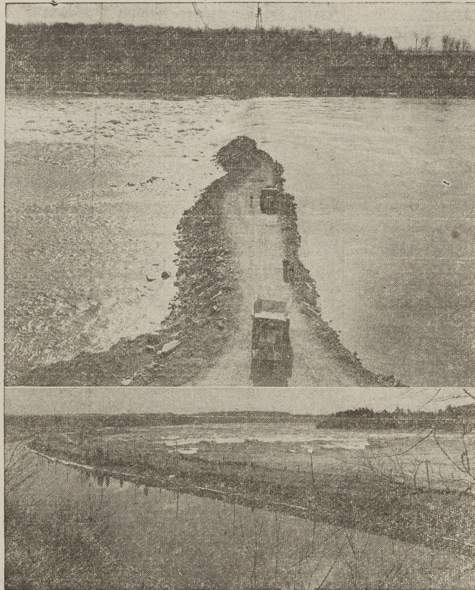
THE LONG SAULT SILENCED — The lower picture shows the famous Long Sault Rapids as they have been for generations. But man has changed the flow pattern down the ancient river bed, and this week cut off the water with a rock-fill cofferdam shown above and diverted the water through a wide excavation in Long Sault Island into the south Channel. The water now pours through the sluices of the first stage of the Long Sault control dam. All this work is being done to dry up the river bed in the area of the Long Sault Rapids to complete the second stage of the permanent Long Sault concrete control dam, so that the curved axis structure can be extended over to the head of Barnhart Island. The Long Sault Rapids have disappeared for all time. —Ontario Hydro Photo
