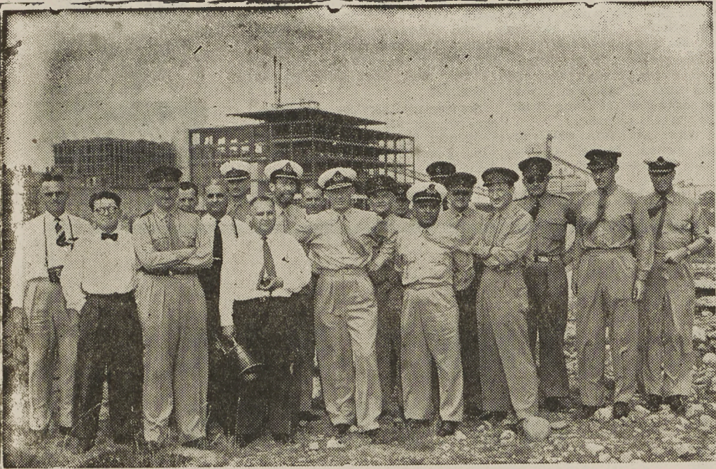
OFFICERS VISIT PROJECT — High ranking officers of the three Services, Army, Navy, and Air Force, who are members of the Imperial Defence College, visited Ontario Hydro St. Lawrence Power Project recently. The group was headed by Admiral D. Crawford. They were taken on a complete tour of the forty mile long project by Information Officer C. G. W. MacIntosh. —Ontario Hydro Photo
