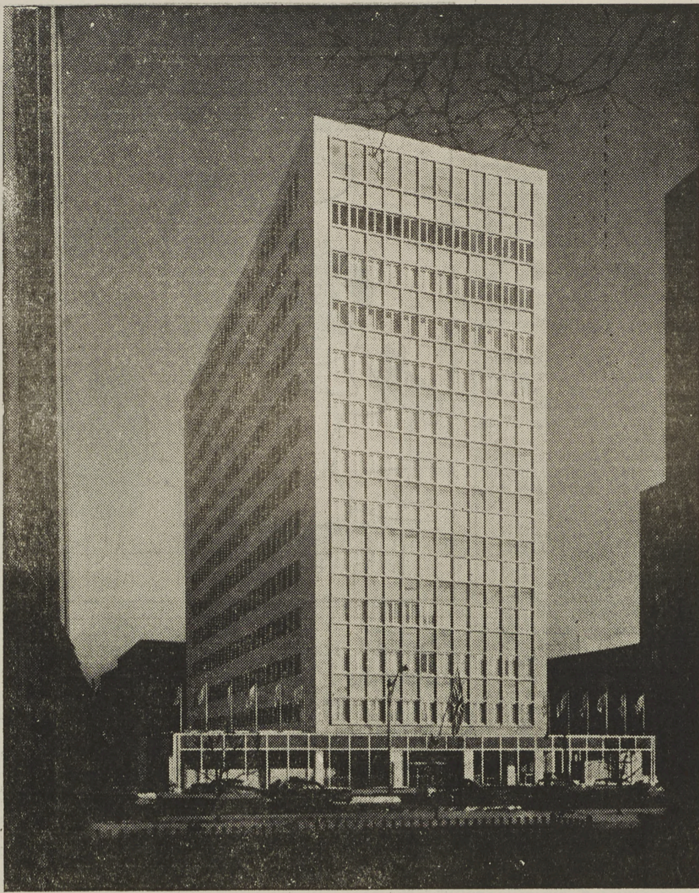
A view of the new $6 million, 13-storey Shell Building, 505 University Avenue, Toronto
